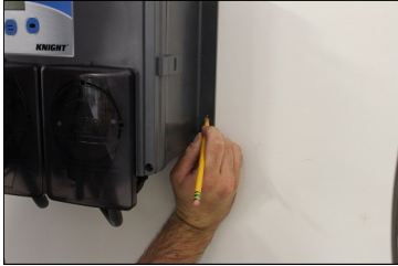
(10) Mark position of lower two keyholes.
