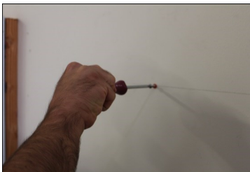
(8) Insert screws into anchors leaving 1/4" space.
