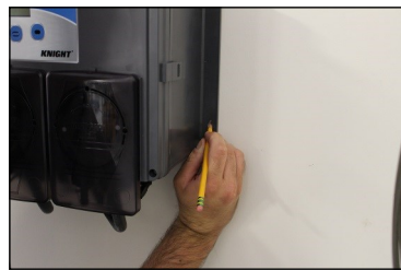
(10) Mark position of lower two keyholes.
