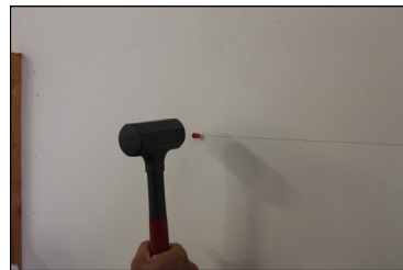
(7) Tap wall anchors into both holes.
