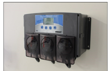
(9) Hang unit on screws through the upper two keyholes.
