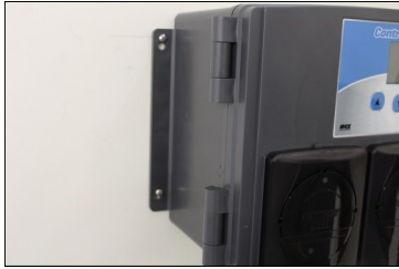
(13) Hang unit and tighten all four mounting screws.
