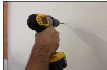
(6) Drill 3/16" holes in the two marked positions.
